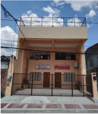
Phase II of the REACH office construction plans will include a second and third floor above the mezzanine.
